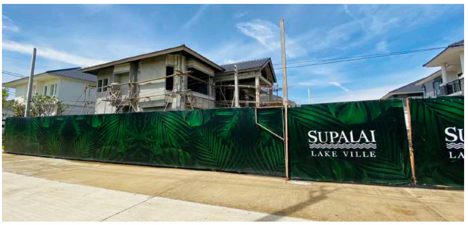
Inspect metal sheet fences
