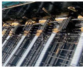
Rubber Former heard are used to replace foam Former heard for the Anchorage head
